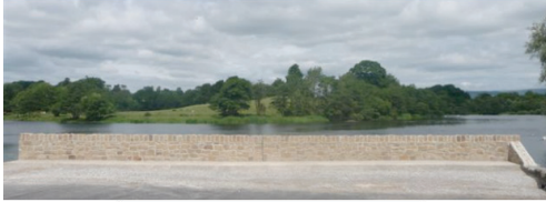
Ferry Car Park Wall
