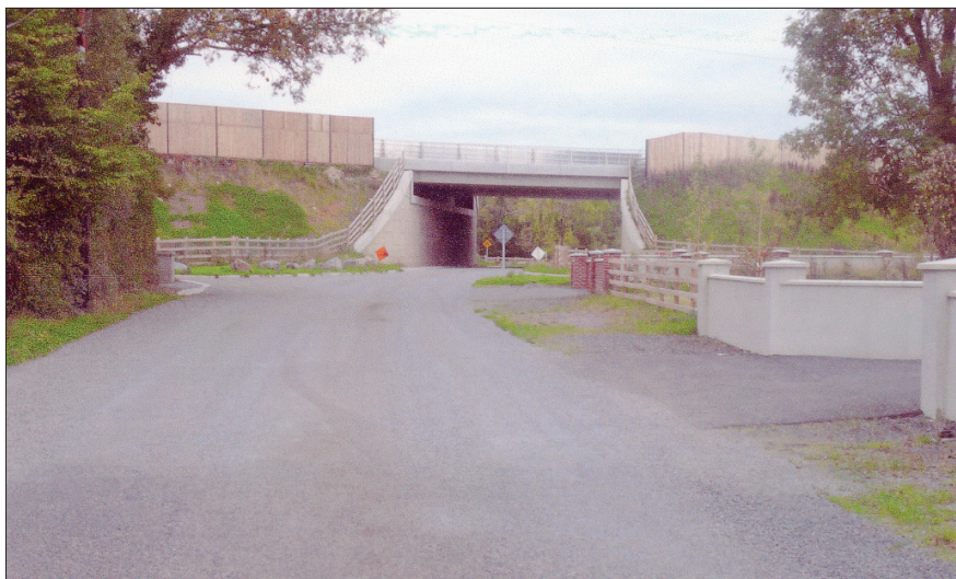
An Caisleán - The Castleconnell, Ahane, Montpelier Annual 2010
